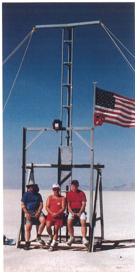
Phil, Paul, and Jim take a break after erecting the tower.
